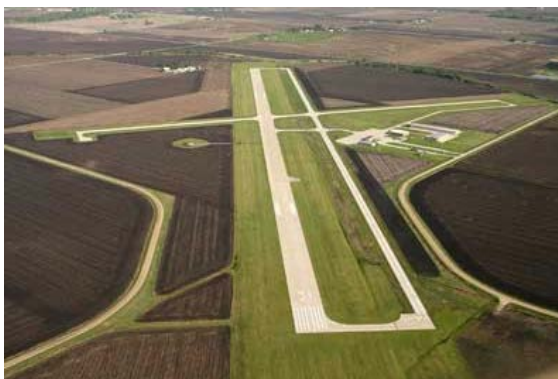
Construction of the taxiway parallel to the main runway was a condition for receiving the new system.
